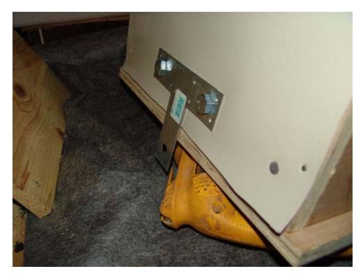
Before you put the screws into the hinge, make sure that the back of the roof is right up against the metal T bracket.
