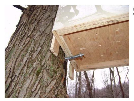
Here is a picture of the bottom hanger bolt installed.
