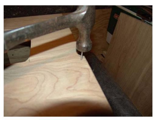
Nail the sides together. The best nails to use are stainless steel ring shanked nails. You can also use galvanized or stainless steel screws.
